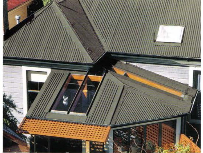
Roof: Resene Mid Grey N55-005-250
