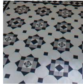
Foyer floor tiles: Winckelmans range from Tile Trends
