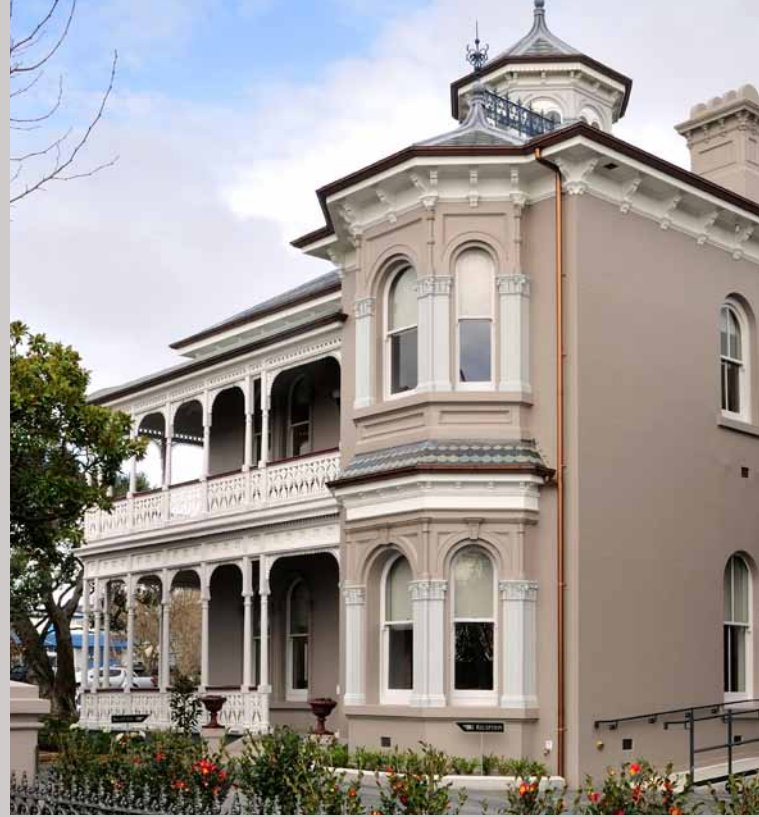
A Heritage Colour Maestro award was won by Peter Reed of Salmund Reed Architects for Allendale House in Auckland. It uses Resene Quarter Oilskin walls, Resene Silver Chalice on the turret, Resene Half Rakaia mouldings, Resene Black White trims and Resene Blast Grey on the fence.
