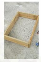
Step four In the same way, fix the second 800mm length and another of the 500mm lengths to form a rectangular frame, as shown.
