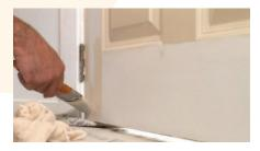
We have chosen not to paint the door hinges, if this were not the case they should be completed last with door almost closed.
