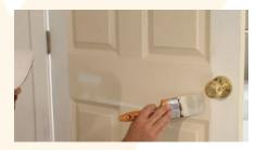
Now complete the outside sections of the door, starting at the base closest to the door hinges and work around the door.
