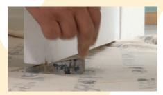
Load the brush with paint – the painter is using a 50mm Legend brush, ideal for use with Resene waterborne enamels.
