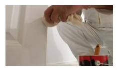
Now paint the internal panels beginning with the rebated edges.
