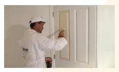
**Note:** The painter lays the paint off as he goes and manipulates the angle of the brush to ensure all areas are covered with minimal brushmarks.
