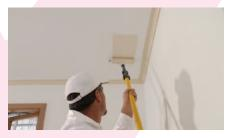
Aim to complete approx 1 m<sup>2</sup> for each roller load (based on using a 230mm PAL No.1 roller sleeve).
