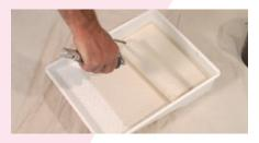
Hold the paint brush as you would a pen the further down the handle the better control you have. By wiping the brush's leading edge on the edge of the paint pot you will cut in more precisely.
