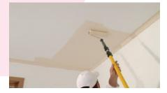
Unlike wall areas ceilings are typically layed-off as the painter progresses. Lay-off each completed section into the previous section.
