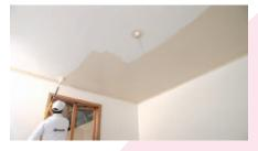
Once the ceiling is complete allow two to four hours to dry and apply a second coat repeating the process.
