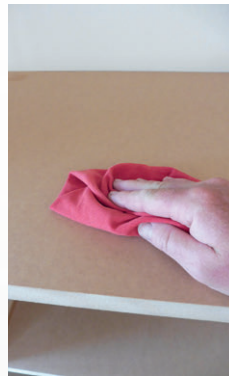
Step three Sand the filler and wipe off any sanding residue with a clean cloth.
