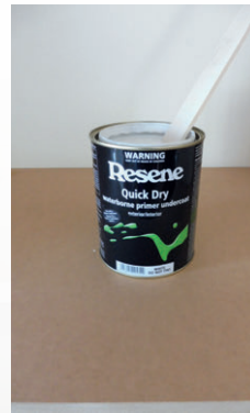
Step four Carefully stir the Resene Quick Dry.
