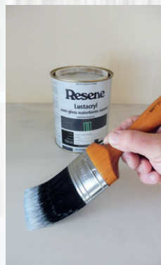
Step seven Apply one coat of Resene Lustacryl tinted to Resene Alabaster to the MDF unit and allow two hours to dry.
