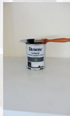
Step eight Apply a second coat of Resene Lustacryl tinted to Resene Alabaster to the MDF unit and allow two hours to dry.
