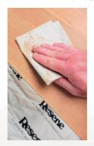
**Step two**Sand the entire table, ensuring any old varnish is completely removed.
