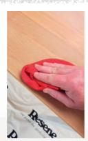
**Step three**Wipe off any sanding residue with a clean cloth.
