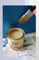
Step eight Apply two coats of Resene Aquaclear gloss to the outside of the cabinet, allowing two hours for each coat to dry.
