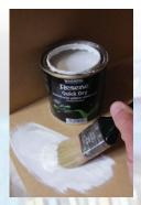
Step two Apply one coat of Resene Quick Dry to the cabinet and allow two hours to dry.
