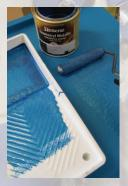
Step seven Apply two coats of Resene Yeehaa to the outside of the cabinet, allowing two hours for each coat to dry.
