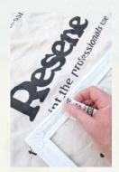
**Step two**Lightly sand the plastic frame to 'key' the surface.
