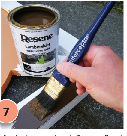
7 Apply two coats of Resene Burnt Umber to the outer frame and inner supports, allowing two hours for each coat to dry.
