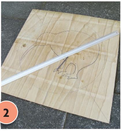
2 Rule a central vertical line, a central horizontal line and diagonal corner-to-corner lines to mark the centre point. Fix one end of the string to the pencil and the other to a thumb tack at the centre point so you can draw a 430mm radius circle.
