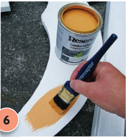
6 Apply two coats of Resene Light Tan to the central circle, allowing two hours for each coat to dry.
