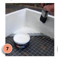
Apply two coats of Resene Alabaster to the larger frame, allowing two hours for each coat to dry.
