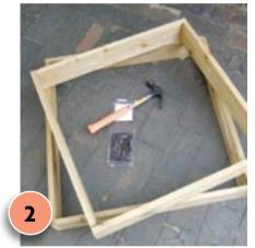
Using PVA glue and galvanised nails, attach the four longer lengths of timber together to create a square frame, checking its shape with a set square. Repeat with the shorter lengths of timber.
