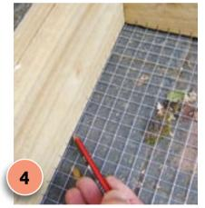
Mark the lines of mesh around the inner edge with a pencil, as shown – make sure the lines of mesh on the smaller frame are halfway between each pencil mark. Remove inner frame. Repeat step 3(a).
