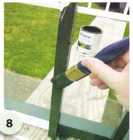
8 Apply two coats of Resene Black Forest to the entire frame, allowing two hours for each coat to dry.
