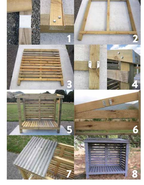
a BACK Lay the posts with the 13° angle facing downwards; 200mm up from the bottom of each, cut a rebate 50mm deep x 100mm wide, undercoat then coach-bolt a lower bar into the rebates. FRONT Lay the posts with the 13° angle facing upwards, repeat the bottom bar procedure. Coach-bolt an upper bar to the outside of the two front posts, about 10mm below the top edge.
