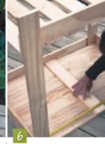
Turn the potting table over and mark the centre. Then screw the last 60cm plank to the underside of the table for extra strength.
