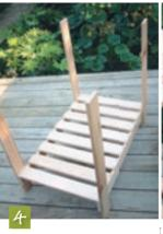
Stand the potting table upright. To create a frame for the top, screw a 60cm plank (held vertically) across each end.
