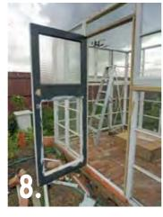
glue. Assemble the roof frame, as shown, with centres of each rafter approximately 600mm apart. Once again, use temporary bracing to keep the frame upright and in position during construction.
