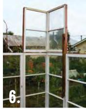
the glasshouse, as shown. Fix at the base with construction glue and 90mm screws, countersinking the screw heads. Again, keep this structure stable with temporary bracing.
