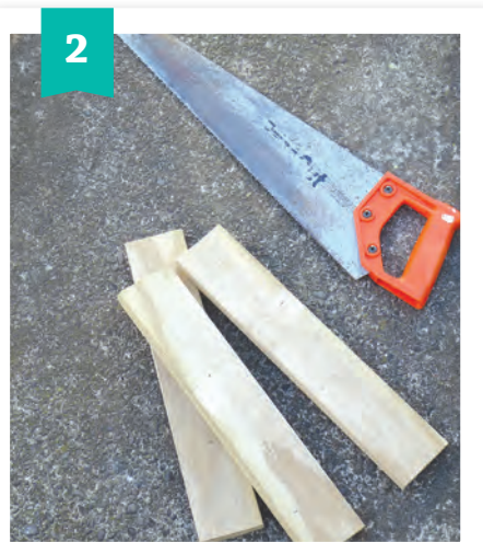
2 Use pencil marks as a guide to cut the fence palings, as shown.
