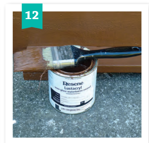
Apply a second coat of Resene Cioccolato to the unit, again allowing two hours to dry. Fix to the fence with 40mm screws.
