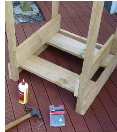
5. Attach two more pieces of fence paling across the base of the composter with PVA glue and nails, and two pieces across either side.
