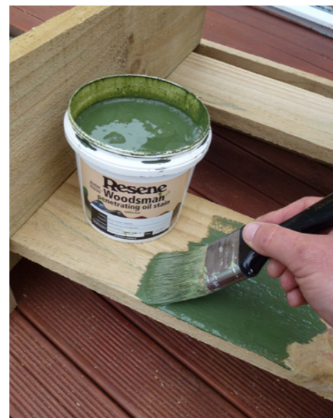
10. Apply two coats of Resene Woodsman to the composter and door frame, allowing 24 hours for each coat to dry.
