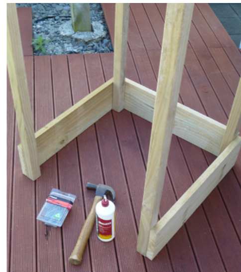
4. Fix two more pieces of fence paling to the remaining 1.1m lengths to form the base of the composter. Again, use the set square to ensure corners are all at right angles.
