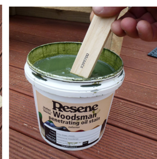
9. Carefully stir the Resene Woodsman with a paint stirrer.
