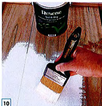
10 Apply one coat of Resene Quick Dry to the entire planter and allow two hours to dry.
