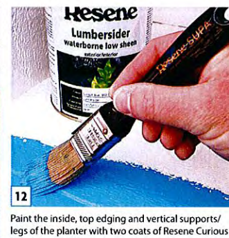
12 Paint the inside, top edging and vertical supports/legs of the planter with two coats of Resene Curious Blue, allowing two hours for each coat to dry. Line the planter with polythene sheeting, fixing at the top edge with galvanised staples. Cut some drainage holes in the polythene at the base of the planter and fill with good quality potting mix (not garden soil).
