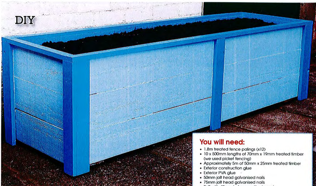
4 Attach two more of the full fence palings along the front and back edges, as shown, and two of the 530mm lengths at either end. Fix firmly with 75mm nails and construction glue.
