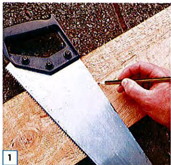
1 Measure and mark six lengths of fence paling at 530mm, and three lengths at 480mm. Use the back of the handsaw, as shown to ensure pencil guide lines are at forty five degrees.
