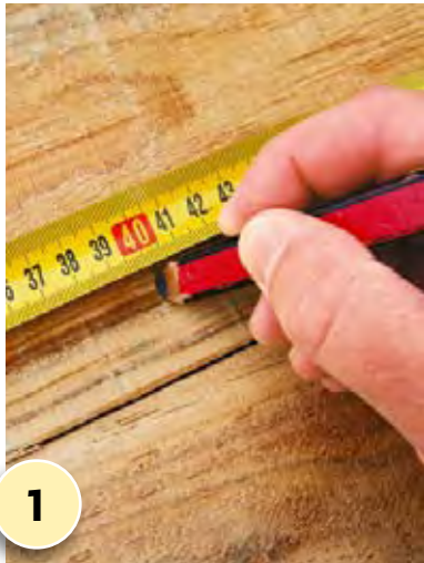
1 Measure, mark and cut four lengths of fence paling 400mm long and three lengths of fence paling 350mm long.
