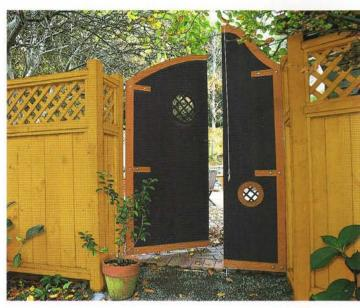
Sharp edges on timber are very difficult to paint as paint tends to flow away from edges leaving weak spots. For best results these sharp edges should be sanded to a rounded profile prior to painting.
