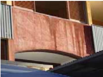
In the case of limewashes they leach lime, an extremely alkaline material that will etch glass and attack aluminium windows. Resene AquaShield is recommended for these projects as it will give a similar looking finish without the unwanted lime leaching. The accompanying photo shows the deterioration of a limewashed building – it is unsightly and particularly obvious with stronger colours.
