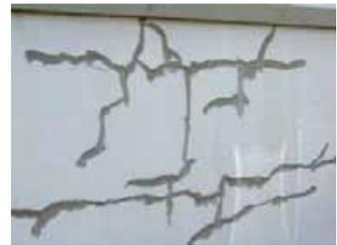
As a rule, most commercial sealants should not be painted over. However most sealants used for minor exterior repairs or for minor jointing and gaps, such as around window frames, are paintable. For example Selleys All Clear and Fosroc's MS Silicone sealant may be painted, once cured. However, always check the manufacturer's recommendation.
