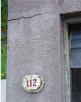
Hairline cracking often occurs as the cementitious surface (usually plaster or render) cures, especially if it is hot or dry, as water in the concrete mixture evaporates quicker than it would normally.
