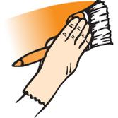
2. When all the wallpaper has been removed allow the wall surface to dry completely, then sand with 100 grit aloe sandpaper to remove all nibs etc and dust the walls. Fill all imperfections with a sandable filler, sand smooth and dust the entire surface then size before hanging your new wallpaper.
