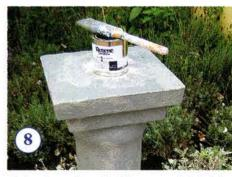
Paint the pedestal with a coat of Quickdry Primer and two coats of Sandtex 'Stack', stippling the second coat for added texture. Position the sundial face on top of the pedestal so that at noon the shadow from the gnomon falls across the XII line (remember to add an hour during daylight saving). Glue the face into position with construction glue.
