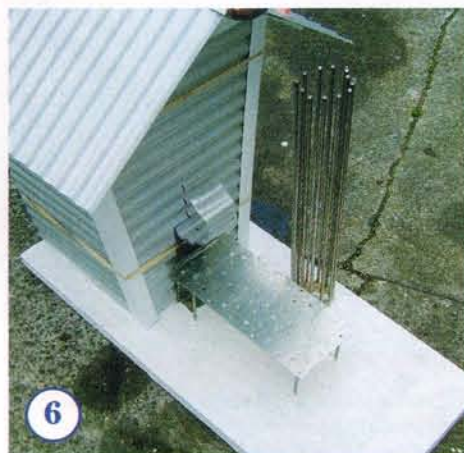
6 MAKE a hole in the top edge of the roof and insert the large screw from beneath. Keep in place with builders' filler. Cut plastic trim to fit front edges and apex of roof. Fix with builders' glue, holding in place with rubber bands until dry. Apply Quickdry Primer to the ply and Galvo One Primer to the Zinalume.
