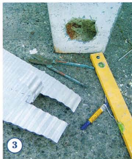
3 WITH the tin snips, cut a hole in the front of the old letterbox. Cut two slits in the front Zinalume panel and curl the centre section up to form the door.
