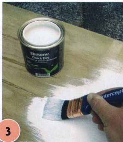
3 Apply one coat of Resene Quick Dry to the entire panel (including side edges and back) and allow to dry for two hours.
