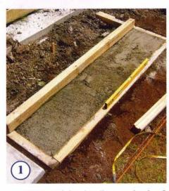
EXCAVATE and level soil to a depth of 100mm and construct a base of (level) wooden shuttering measuring 1500mm x 350mm. Pour 2 1/2 bags of mixed concrete into shuttering, embedding the reinforcing rods for strength. Level the concrete with a long wooden post.
