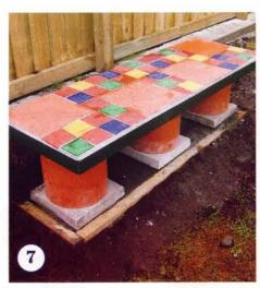
CUT the tanalised wood trim and attach to the edge of the bench with construction glue and masonry nails. Prime, then paint with dark green exterior paint.
