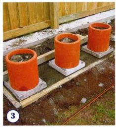
PLACE the terracotta pipes on top of the concrete pavers and fill the base of each one using the remaining half bag of concrete. Fill the pipes with stones or sand to 50mm below the rim.
