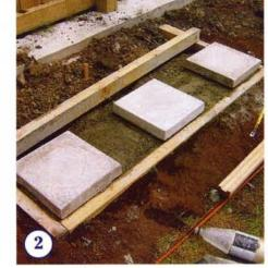
USING the builder's plaster mix, cement the three 300mm x 300mm concrete pavers to the concrete base. Ensure the pavers are level.
