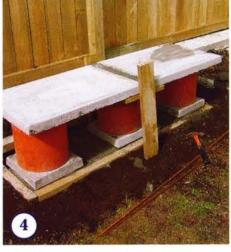
FILL the remainder of each pipe with builder's plaster mix and cement the two 500mm x 750mm concrete slabs into place to form the seat, leaving a central gap of 50mm. Fill this with the rest of the plaster mix, using scrap wood for additional support.
