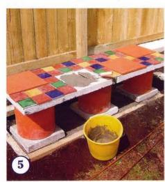
ONCE the cement is dry, remove the wooden supports and lay out the tiles in your chosen design. Using cement tile adhesive, attach your tiles to the concrete plinth.
