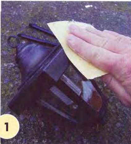
1 Lightly sand the top and base of the light to provide a key for the paint.
