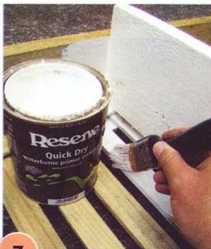
7 Apply one coat of Resene Quick Dry to the shelf unit, allowing two hours to dry.
