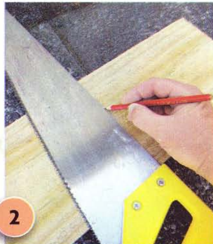
2 Use the saw, as shown, to rule a ninety degree line across the fence paling and cut along this line with the saw.
