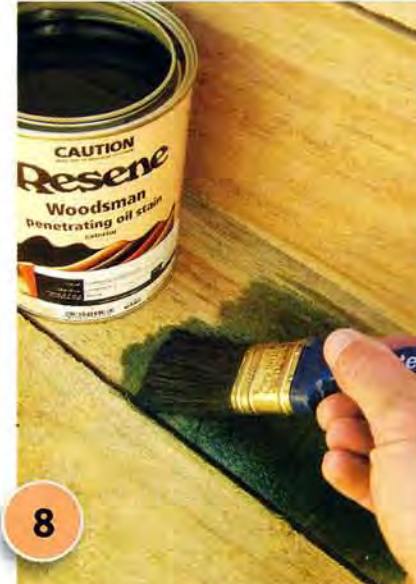
8 Apply two coats of Resene Earthsong to the planter, allowing 24hrs for each coat to dry.
