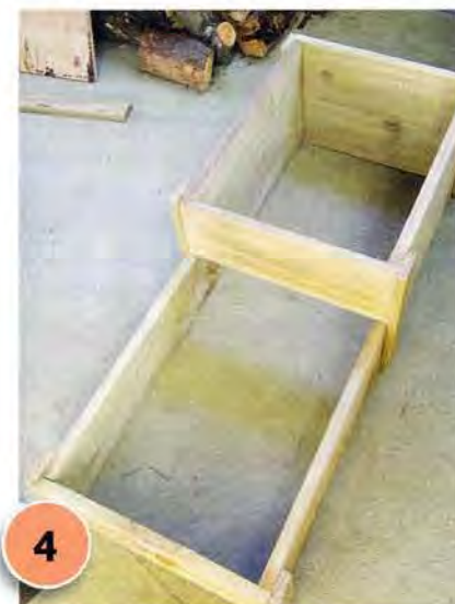
4 Attach the remaining four lengths of rough sawn paling to each of the sides – to create a 'two tiered' box (as shown). Fix together with nails and glue.
