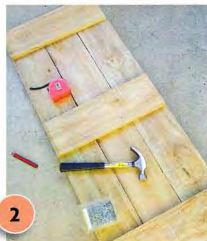
2 Attach three of the 1200mm lengths of rough sawn fence palings together, using three of the 465mm lengths as cross supports (as shown). Fix with 50mm galvanised nails and PVA or construction glue.
